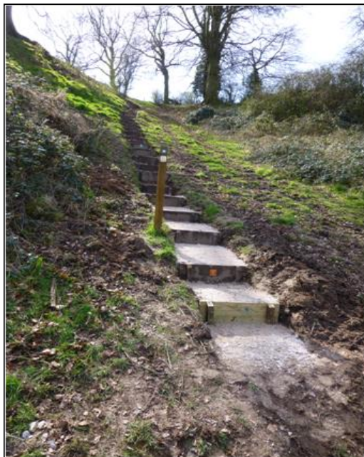
Stoning of steps in progress
